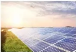
Energy Storage System
