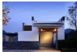
Household Energy Storage
