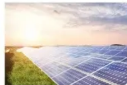
Energy Storage System
